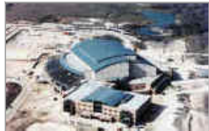
Prestonwood Baptist's 7,000-seat sanctuary and classroom space under construction
